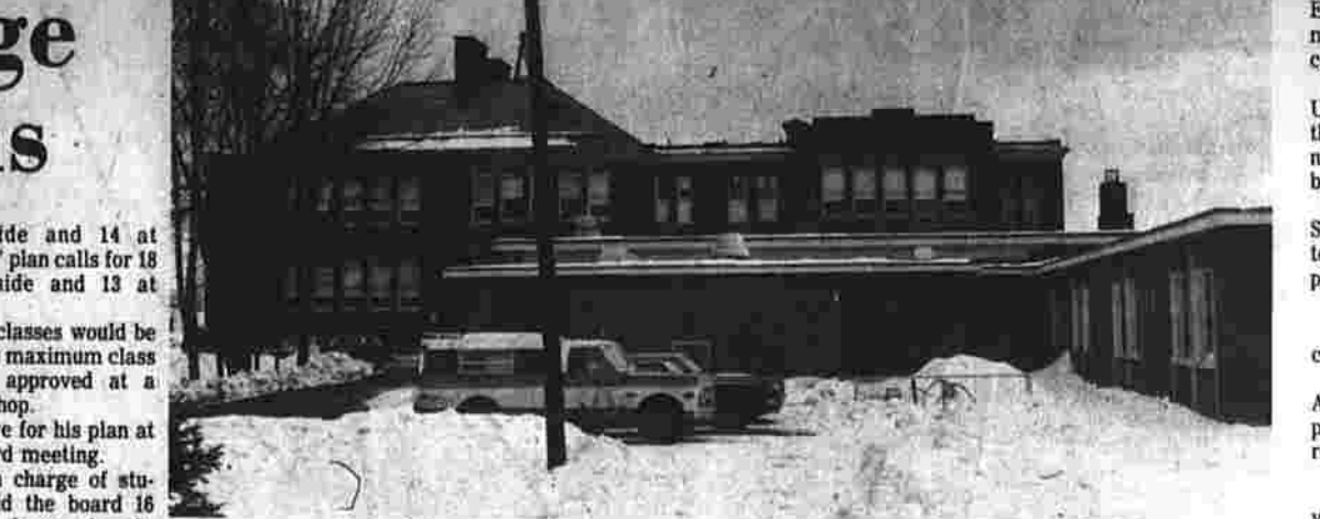
The Burnside School is a combination of old and new. The two-story section was built in 1915. The newer section was added when student enrollment in East Hartford rose to 12,000. It is now below 10,000. The school was recently remodeled inside. Many parents of Woodland School students refuse to send their children to Burnside in the fall despite the closing of Woodland. Many have asked that their children be sent to the town's newest school, Langford. (Herald photo by Barlow)
